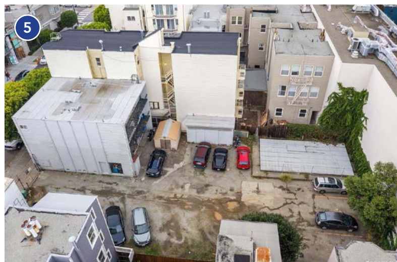
REAR VIEW OF ADJACENT PROPERTIES, NORTH
