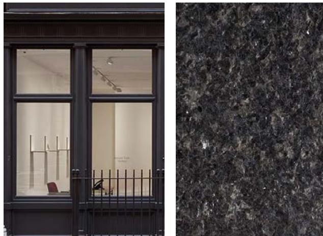
STOREFRONT SYSTEM WITH NONREFLECTIVE GLASS AND GRANITE BULKHEADS
